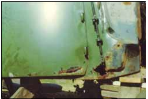
Rust in driver's side door and panel. Note all that existed of six wheel equipment.
