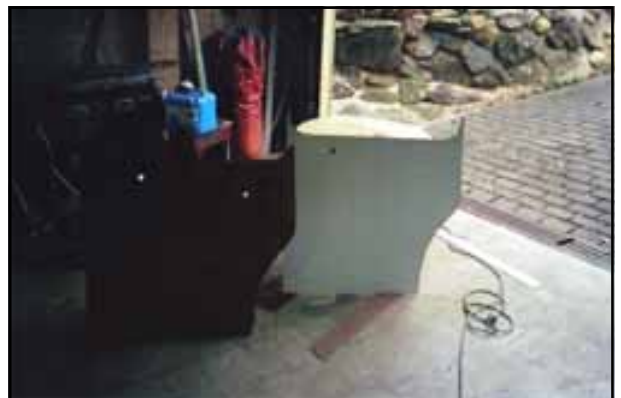
Making of inside door panels
