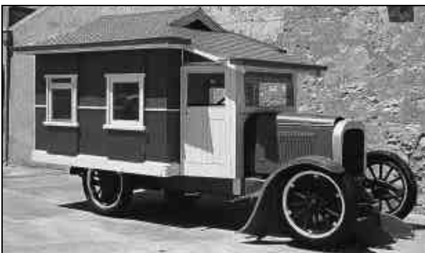
The original Mobile Home at Goolwa.
